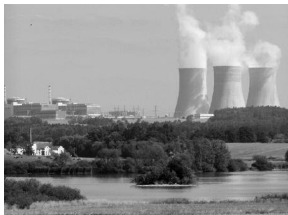
Fig. No 1: Nuclear power plant Temelín is a new landscape landmark in South Bohemia (photo M. Bartoš).
